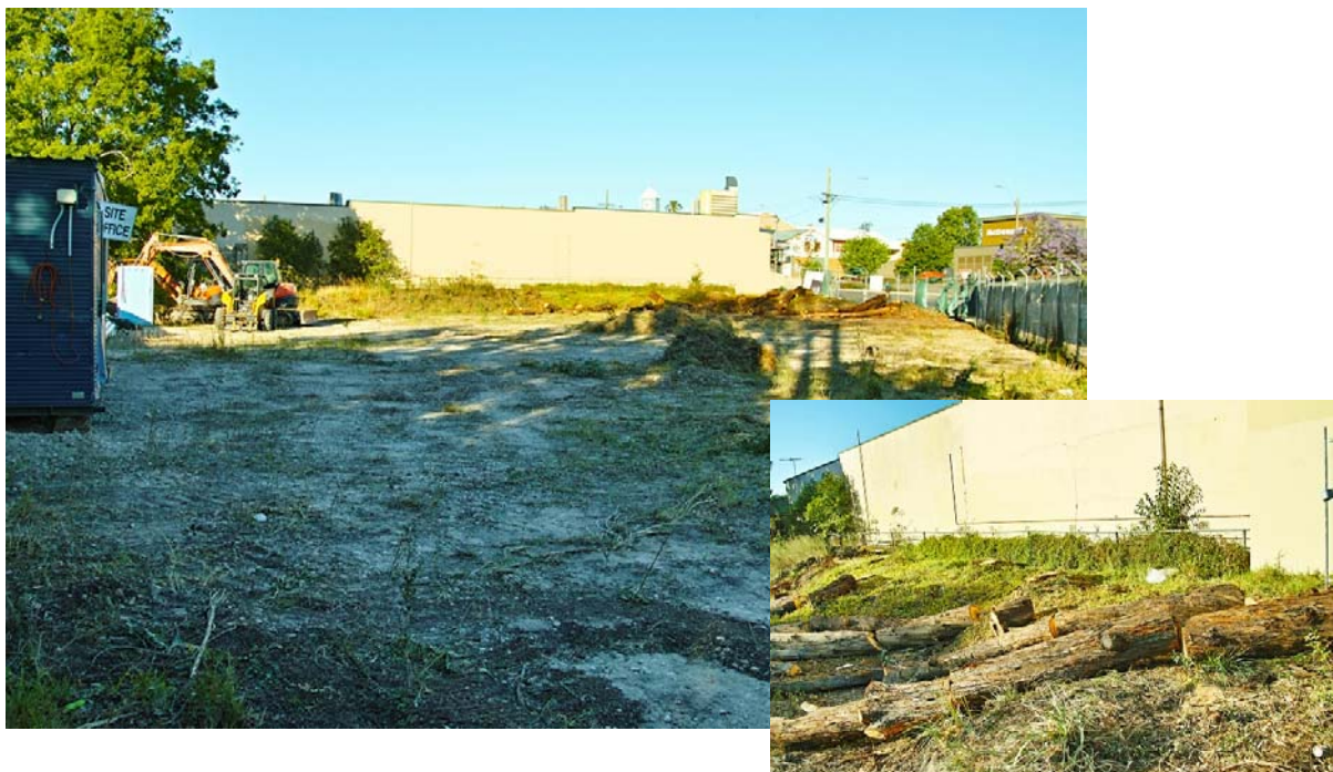
Photos 13 November 2019: Work has commenced.
