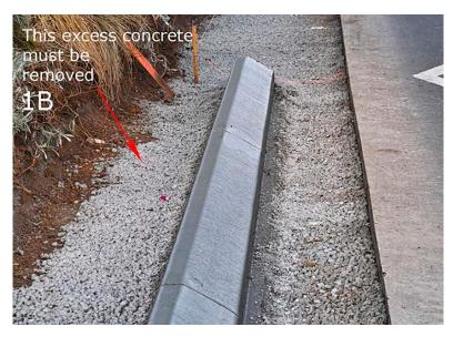
use a concrete saw to remove the excess width of concrete.
