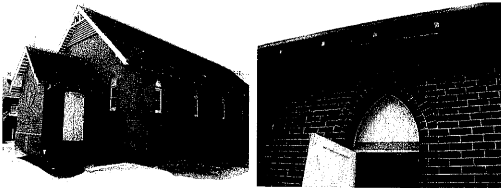
Figure 8 – Church Hall, West Elevation (left) and view of the western wall showing the cracking in the brickwork above the arched door entry (right). The structural cracking has been alleviated by connecting downpipe to water mains to reduce moisture affecting soil conditions under the building (Source: NBRS+PARTNERS, October 2010)
