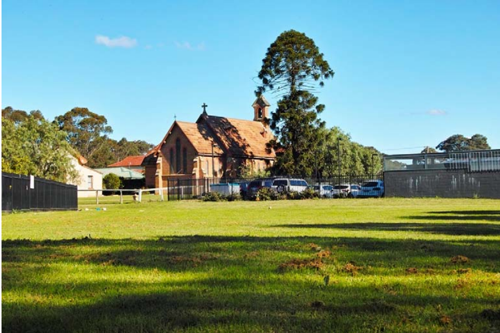
Photos taken from the corner of Camden Valley Way and Richardson Road. The Police station is to the right.
